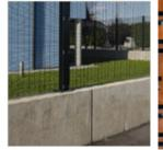
Welded wire fabric fence with board form concrete base
